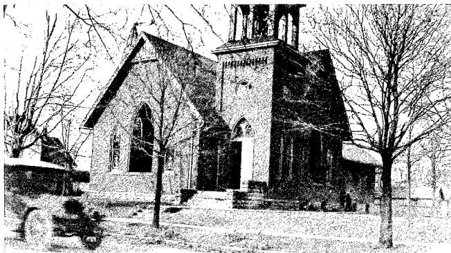
Windows blown out of the Methodist Church.
