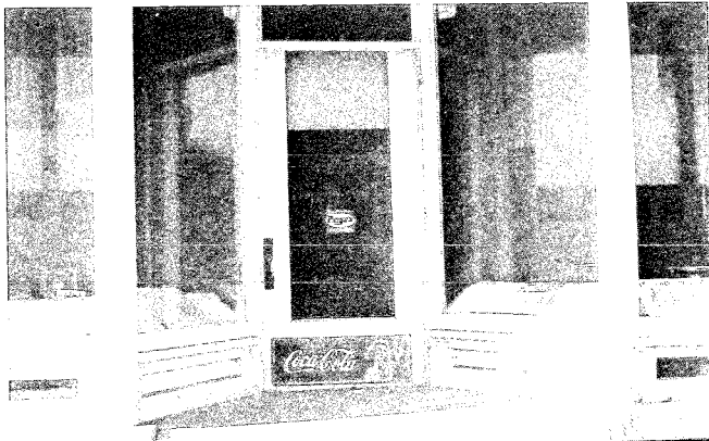
Grove store being renovated
