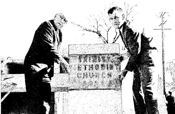
Laying the cornerstone, October 23, 1966. The Rev. I. C. Wynn and Pastor Ben Edwards.
