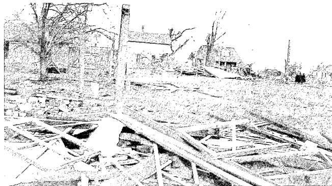
Drennan's house — or what was left — is in the foreground.
